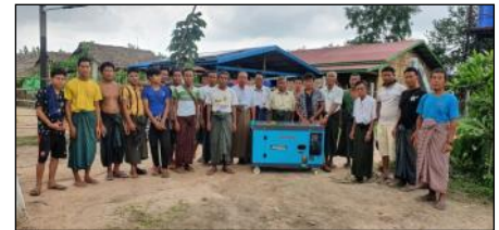
New electric generator for the camp
