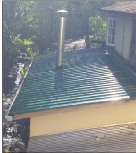
The new roof after installation
