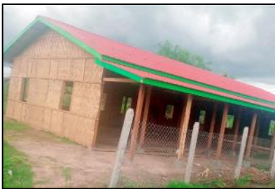
New temporary school building for the children living in the IDP Camp
