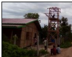
New water tower for the new well
