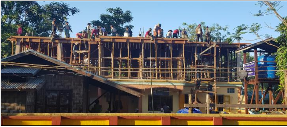
Second floor construction is going on right now at the NPH
