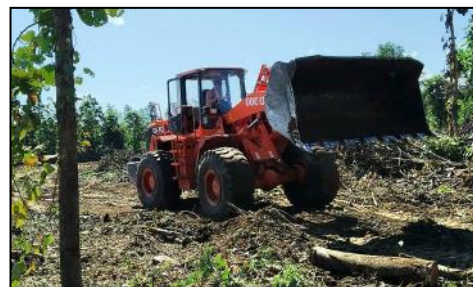
The bulldozer clearing out logs and brush
