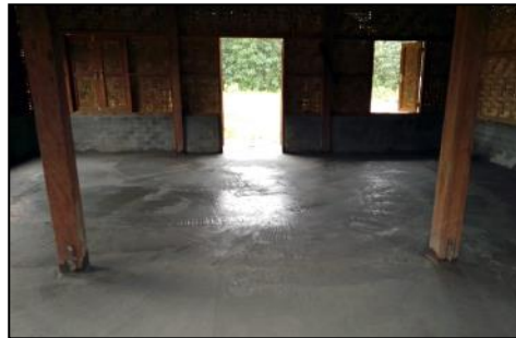
Putting a concrete floor in the new barn
