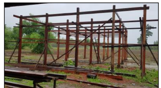
New barn under construction
