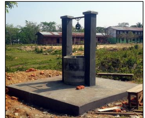
A recently completed well
