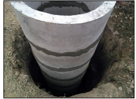
A new well showing the concrete sleeves
