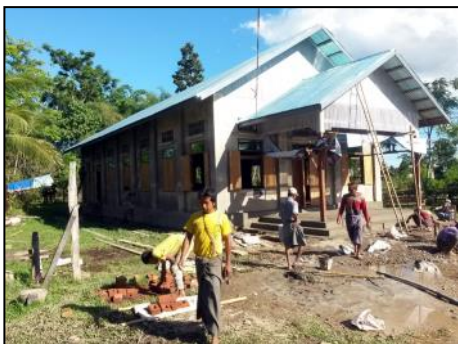
The nearly-completed Lallim Church
