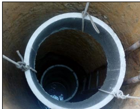
New well under construction
