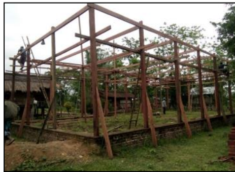
Initial construction of Lallim Church
