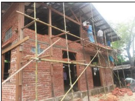
Brick walls going up on Valpabung South
