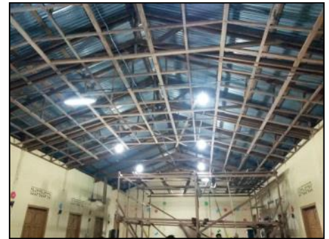
Namihan Church installing a ceiling
