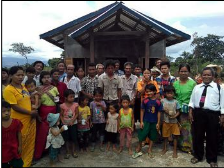
The congregation of Jagnoi Christian Church is very happy with their new brick, concrete and steel building.
