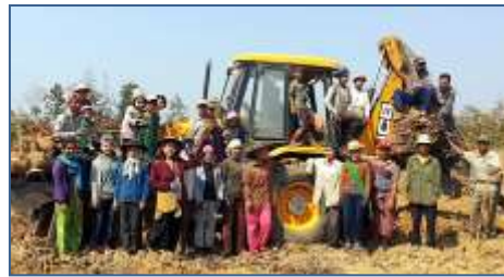
One of the work crews
