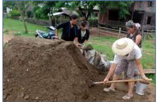
Women of Canaan Christian Church helping with the construction
