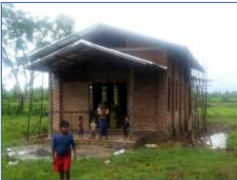
Tingkaya Christian Church (now finished)
