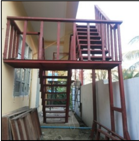
New fire escape under construction
